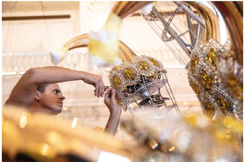
Lapp supplied nearly 7,000 Epic connectors for the installation, including pre-assembled Epic Sensor M12 connectors with stainless steel knurl for connecting sensors and actuators.
