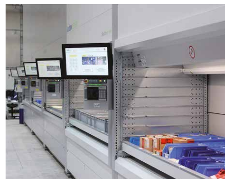
Fig. 1 Kiefel stores up to 14,000 parts in 12 high-bay towers.
