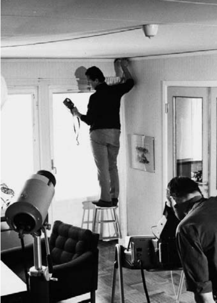
Thermovision 680 performing building diagnostics in Swedish home early 1970s
