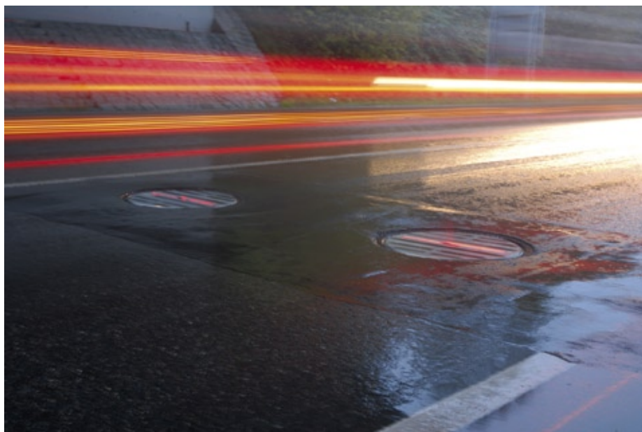
Operation of the ProContour H3D system on federal highway B34 near the company's headquarter in Waldshut-Tiengen, Germany
