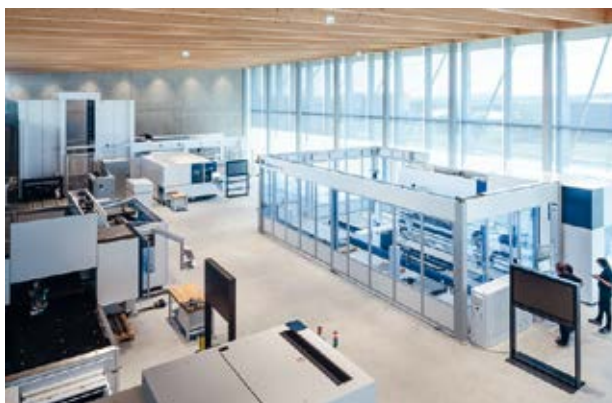
The two-floor building combines offices, seminar rooms, storage areas, a canteen and a demo production unit. (Source: Trumpf)
