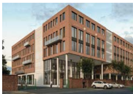
The iWerkx on the Hoepfner site in Karlsruhe, Germany. (Source: PI)
