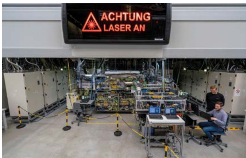
Commissioning of a Trumpf EUV laser system in a so-called installation bay
