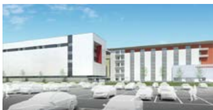
Joko plant 'Building 5' (Source: Hamamatsu)
