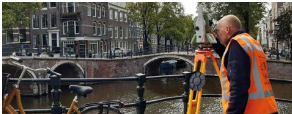
Monitoring of bridges and quay walls in Amsterdam, The Netherlands (Source: Fugro)
