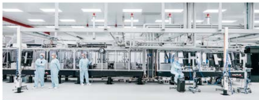
The L3-HAPLS laser system represents a new generation of diode-pumped, high-energy and high-peak-power laser systems. (Source: ELI)
