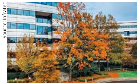
Source: Infratec Infratec Infrared LLC, Office Atlanta, Georgia
