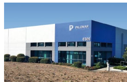
The new headquarters in Carlsbad, CA. (Source: Palomar Technologies)
